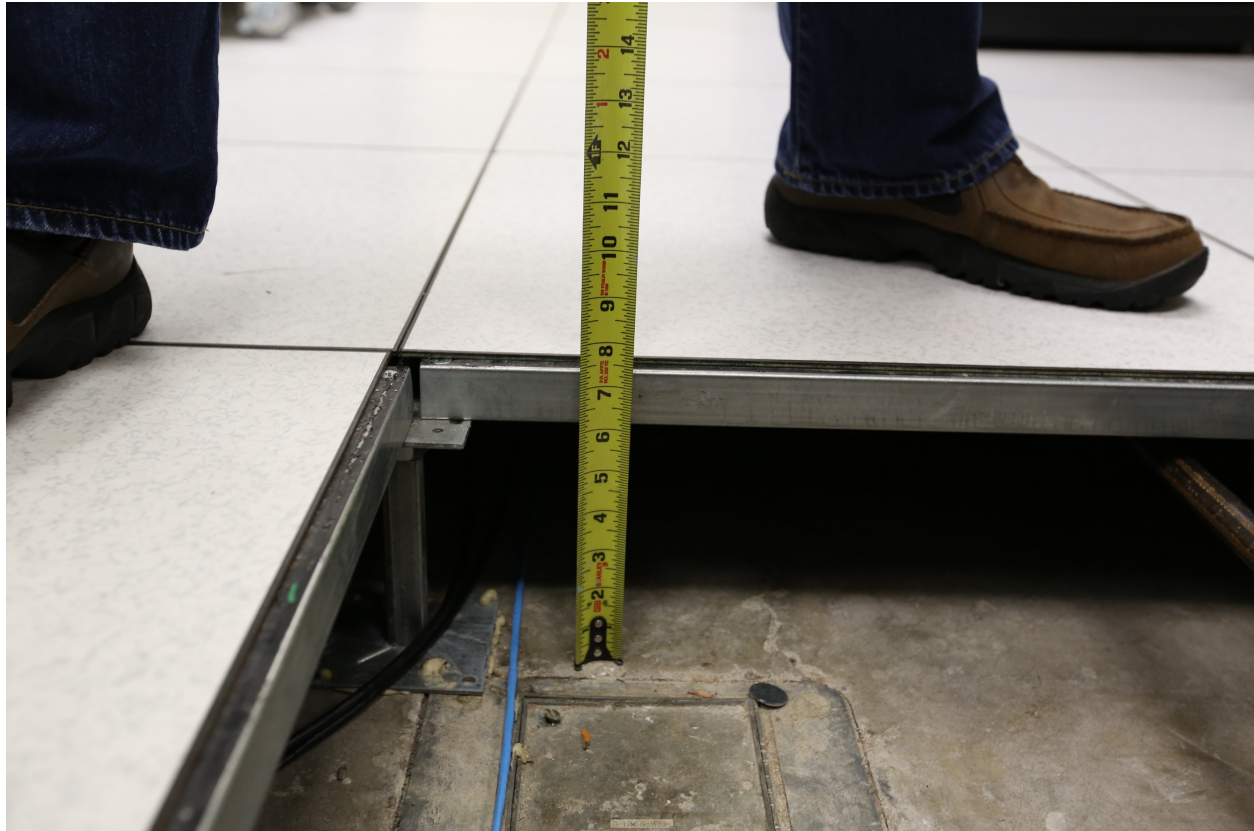
Picture 6. Raised Floor Depth
