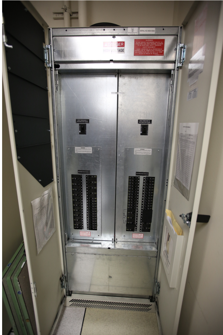
Picture 8. MGE PMM Panel with no labeling
