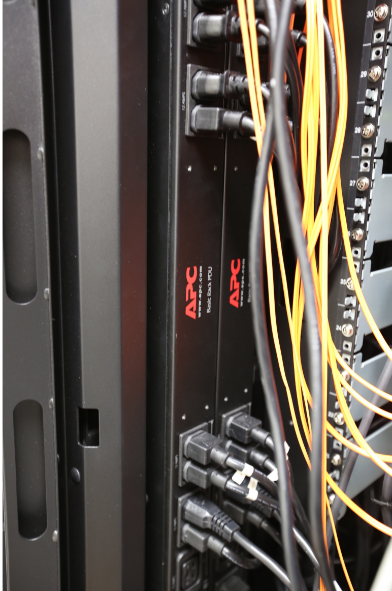
Picture 11. Zero U rack PDU
