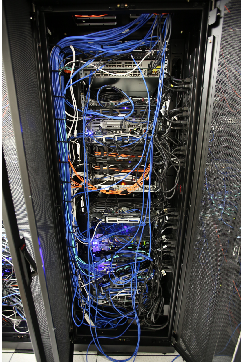
Picture 10. Wiring at back of rack - Restricts air flow
